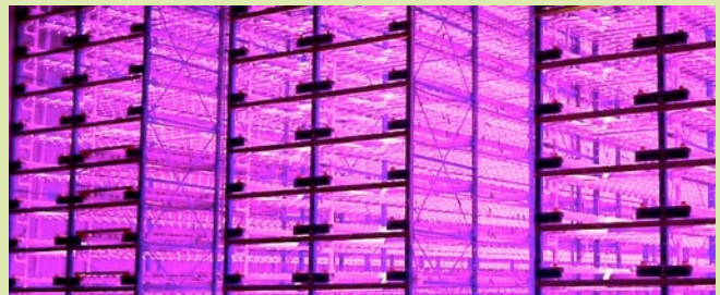
Germination room with produce growing racks with LED lighting in the optimal blue and far red spectra for most plants. (Texas, USA)
